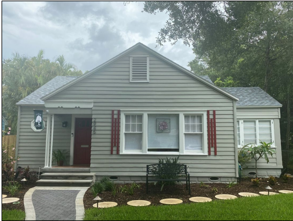
Figure 1: Subject property from 7 th Ave. N.
